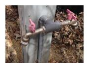
Missing Backflow Prevention on Sanitary Station Water Hose
