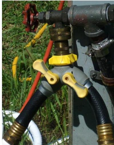
**Answer-** After consulting with the Plumbing Section of the Department of Safety and Professional Services (DSPS), the answer to the question is that a backflow device is to be located on the water supply line hose bib and the splitter(s) needs to be removed.
